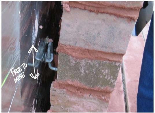
We need to make sure that the anchor is properly placed in the wall so that the tie wire are able to accommodate the up & down movement.
