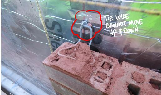
The placement of the wire tie in the wall anchor will impede the movement <u>if misplaced</u> (as shown in the photo above) and cause cracking in the wall.
